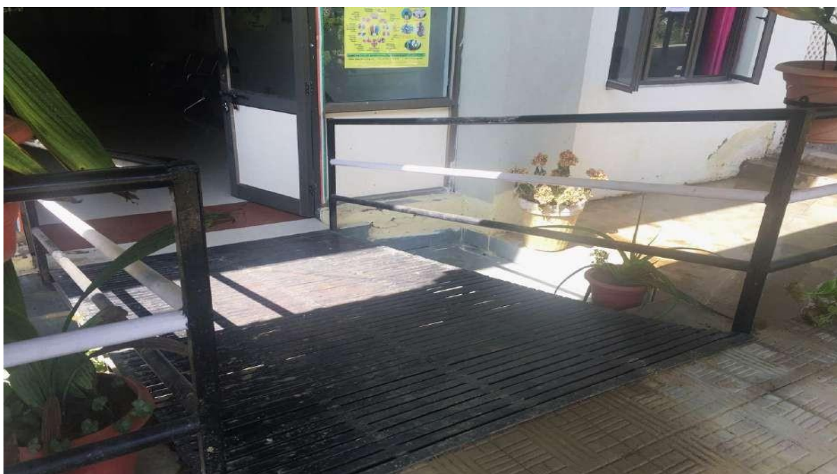
Barrier free access to the administrative block
