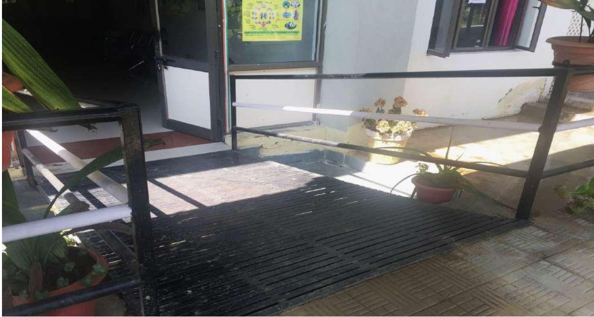
Barrier free access to the administrative block
