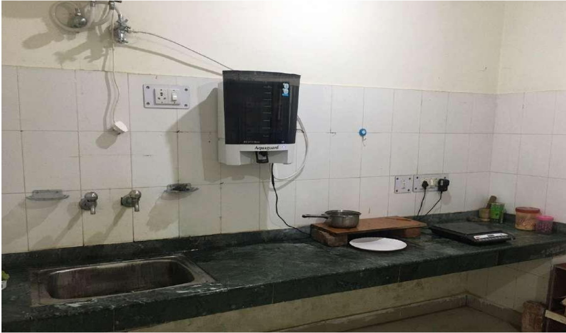
Pantry along with RO water facility for Staff
